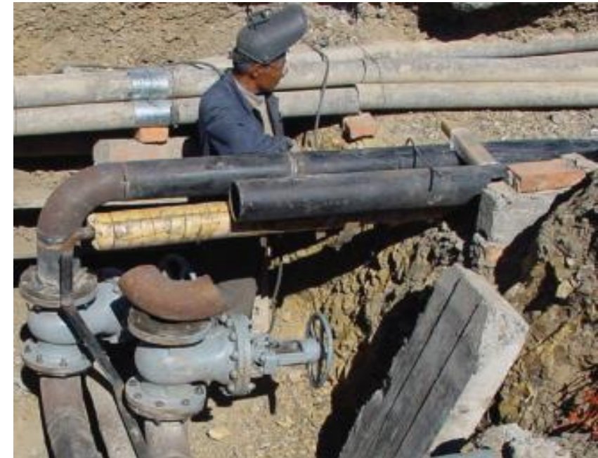
Figure-19: Manually excavated trench
