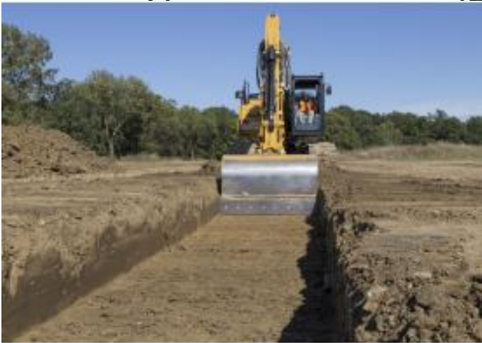
Figure-12: Excavator for wide trench
