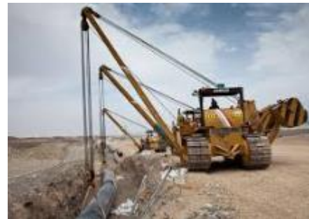
Figure 28: Pipe layer machine
