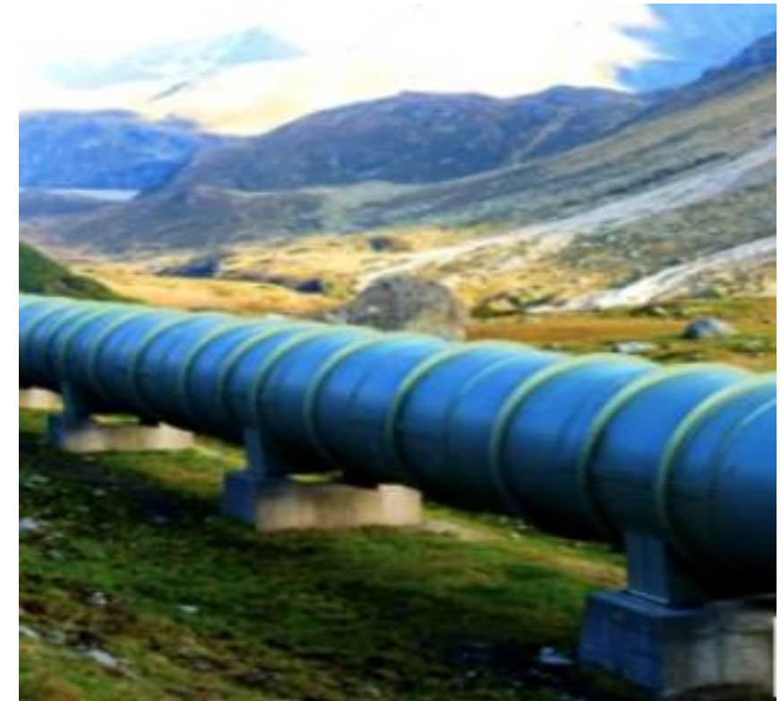
Figure-30: Pipes laid above ground and at crossing ( Bridge attached) and at high slope .
