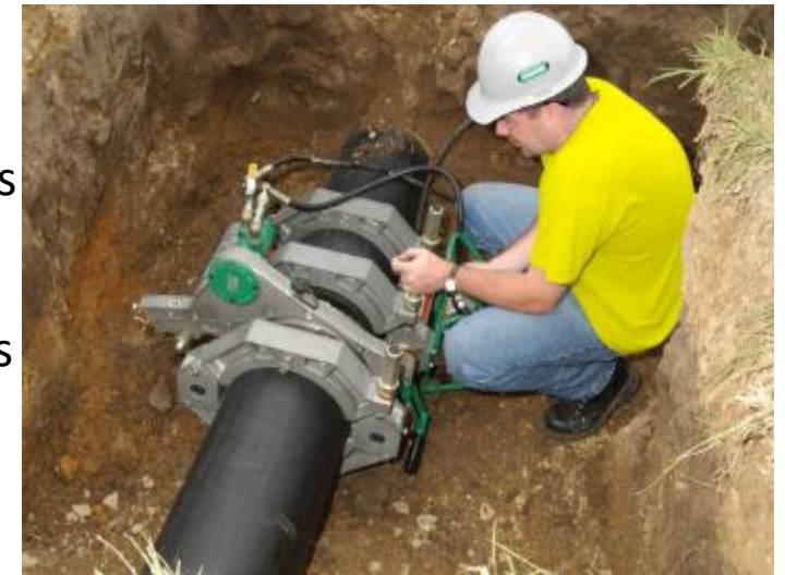
Figure-25: P.E Heat Fusion technique
