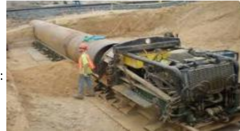
Figure-26: Auger Boring method to cross railway
