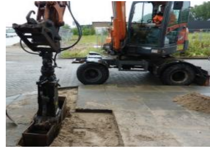
Figure-13: Excavator for narrow trench
