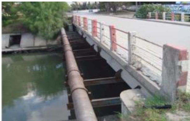
Figure-30: Pipes laid above ground and at crossing ( Bridge attached) and at high slope .
