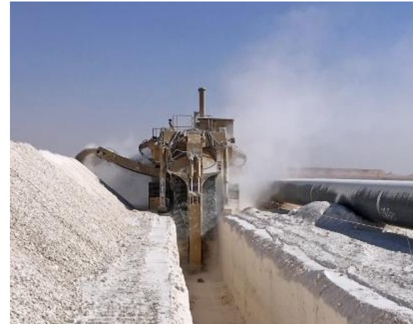
Figure 17: Chainsaw Trencher for big diameter and deep trench 1.8 m ( Courtesy Tesmec)
