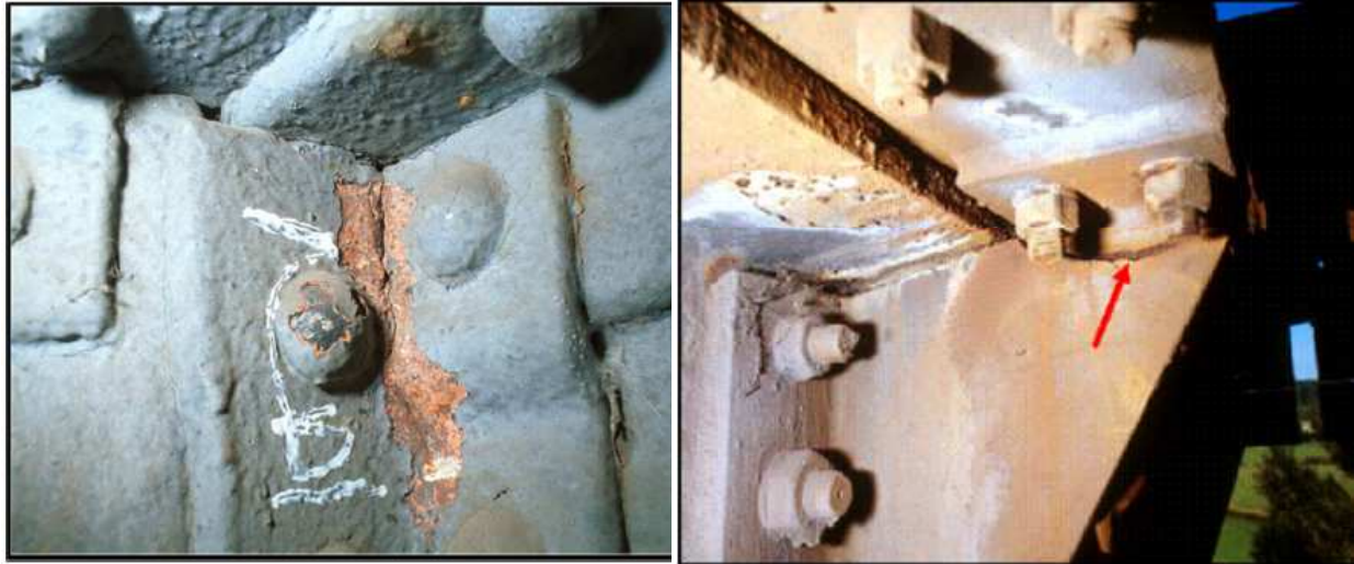
Figure II.4: Fissure de fatigue
