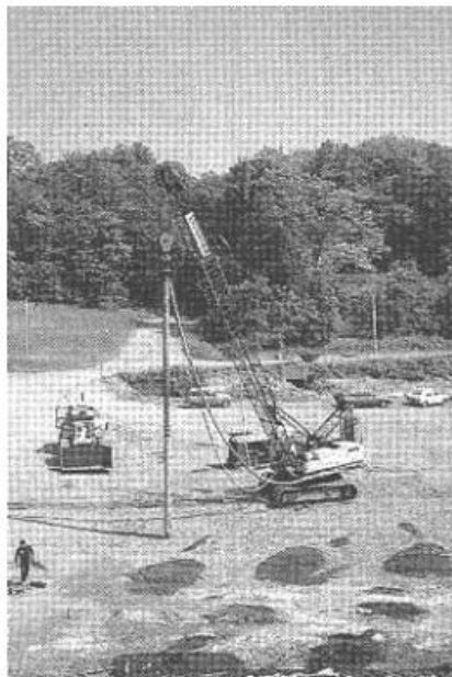
Figure 20 – Chantier de vibrocompactage
