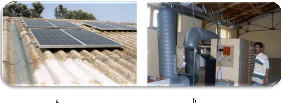
Figure 17. Energy sources of a hybrid dryer: (a) photovoltaic panels and (b) auxiliary diesel-powered energy source (Ouaouich and Chimi, 2005).
